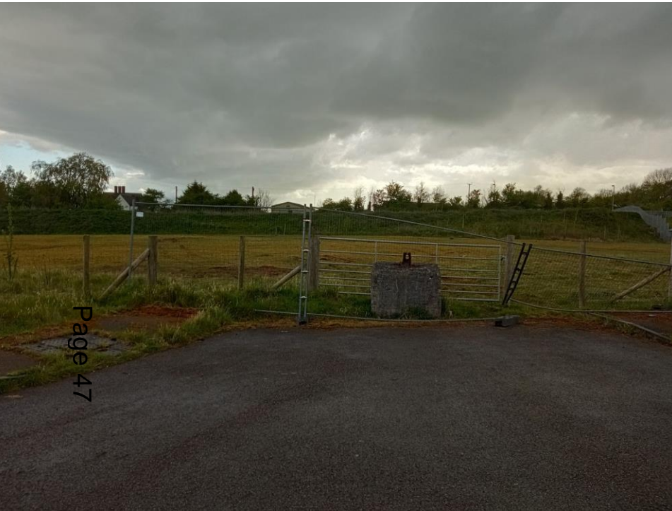
Site access from Buntsford Drive
